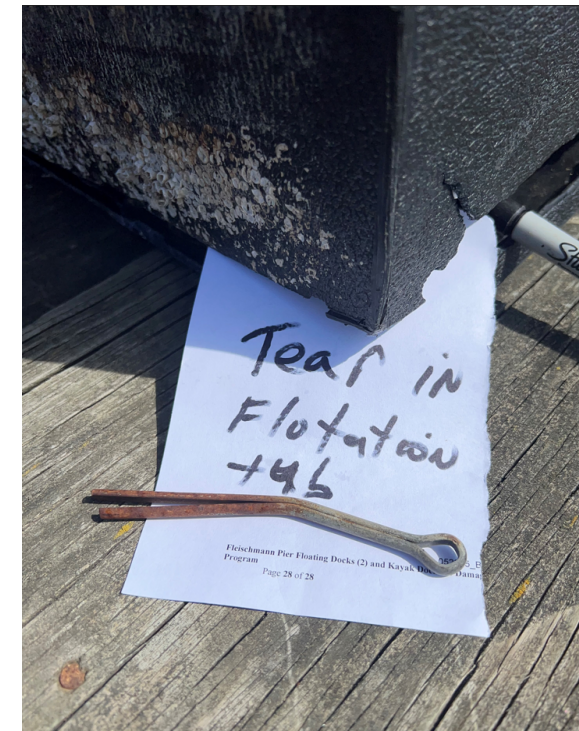
EXHIBIT E.4 TEAR IN EXISTING DOCK FLOAT TO BE REPAIRED W/ 6" DUCK TAPE
