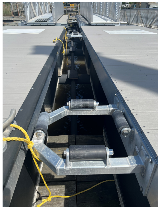
EXHIBIT E.3 EXISTING PILING HOOPS TO BE REMOVED AND REPLACED
