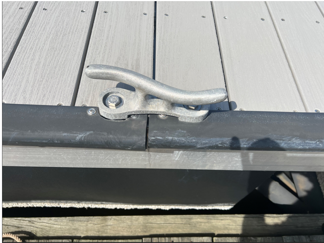
EXHIBIT E.1 EXISTING "S-SHAPED" MOORING CLEAT
