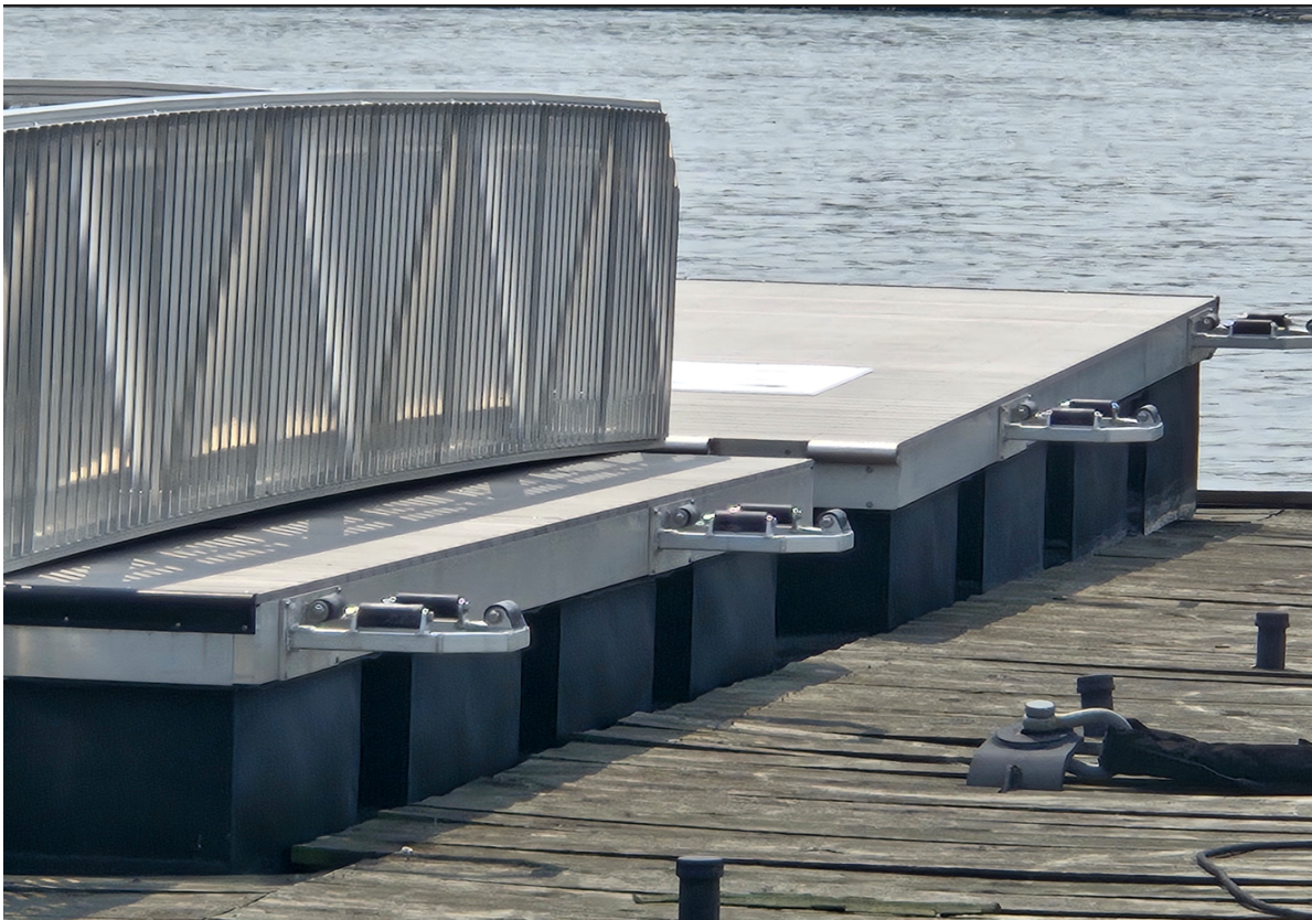
EXHIBIT E.6 AREAS OF FLOATING DOCK TO RECEIVE RUBBER BUMPERS
