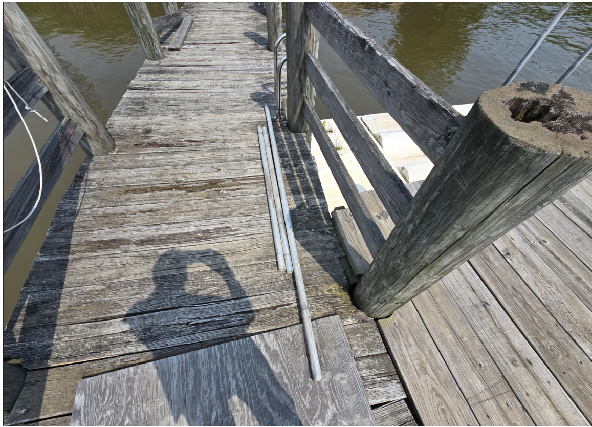
EXHIBIT E.5 PINS FOR INSTALLATION OF FLOATING DOCKS
